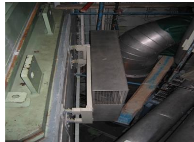
Passive catalytic hydrogen recombiners at operating VVER
