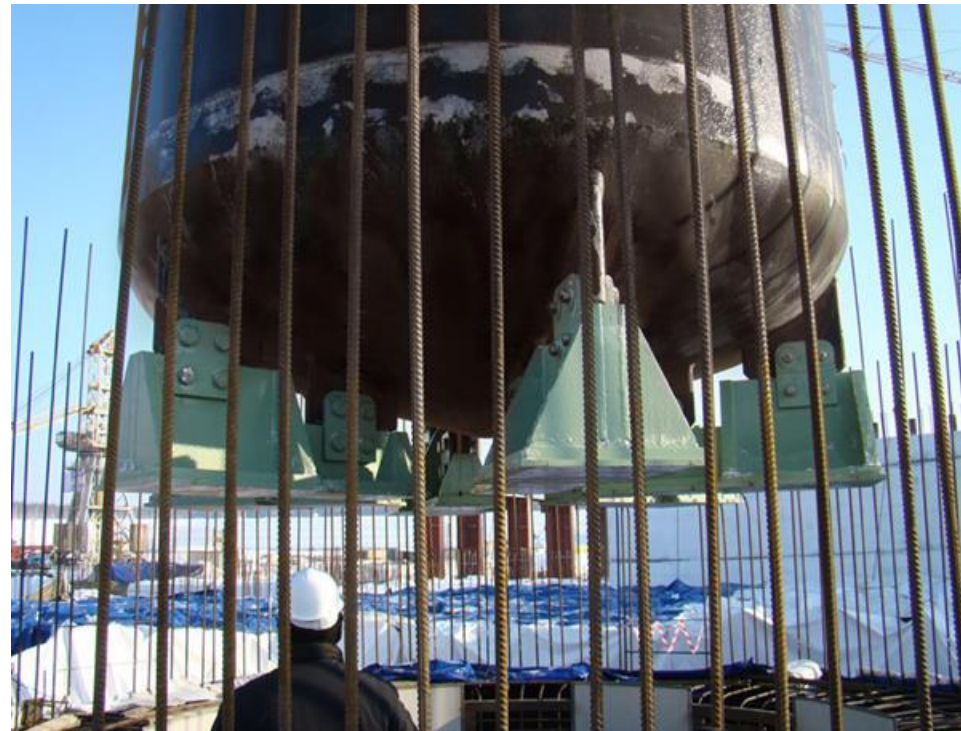
Installation of the shell of the core catcher
