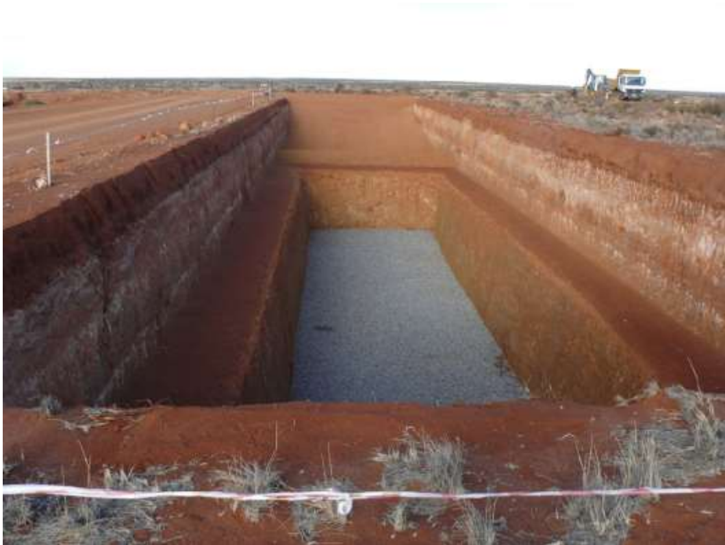
Figure 2: LLW disposal trench at Vaalputs
