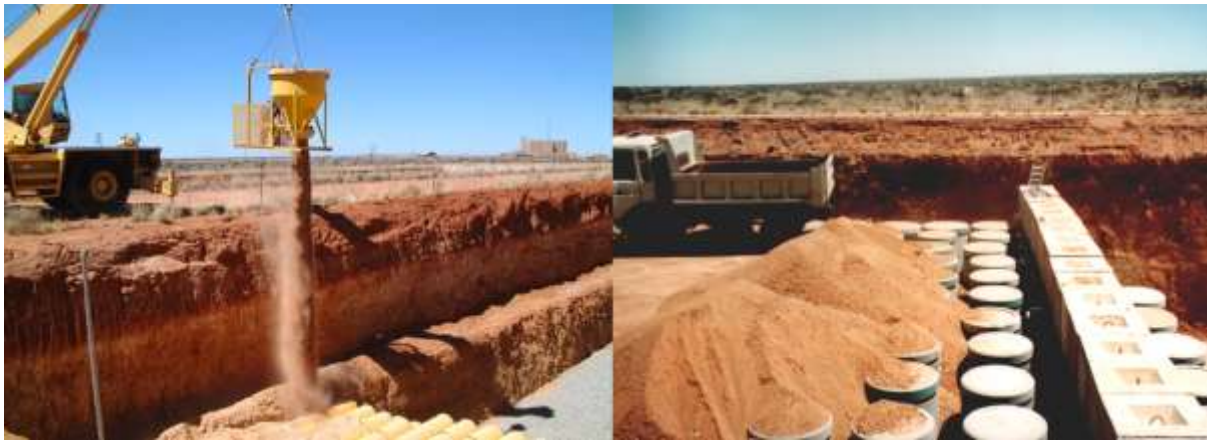
Figure 7: Backfilling of waste packages
