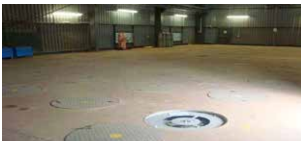
Figure 8: Thabana Pipe Storage Facility
