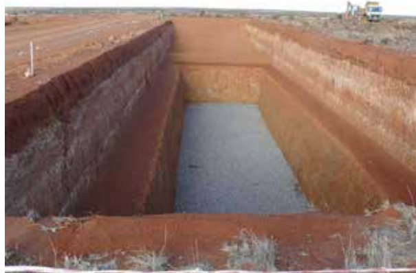
Figure 15: New disposal trench
