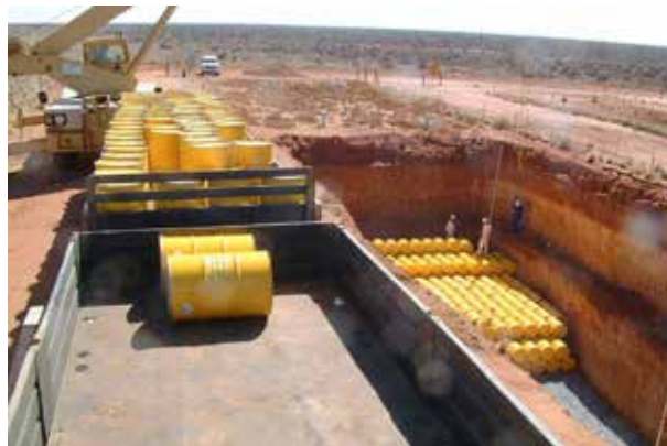
Figure 14: Metal drums being emplaced in disposal trench
