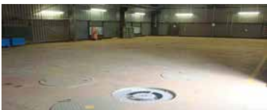
Figure 11: Thabana Pipe Storage Facility
