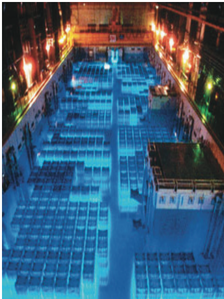
Figure 2: Koeberg Used Fuel Pool
