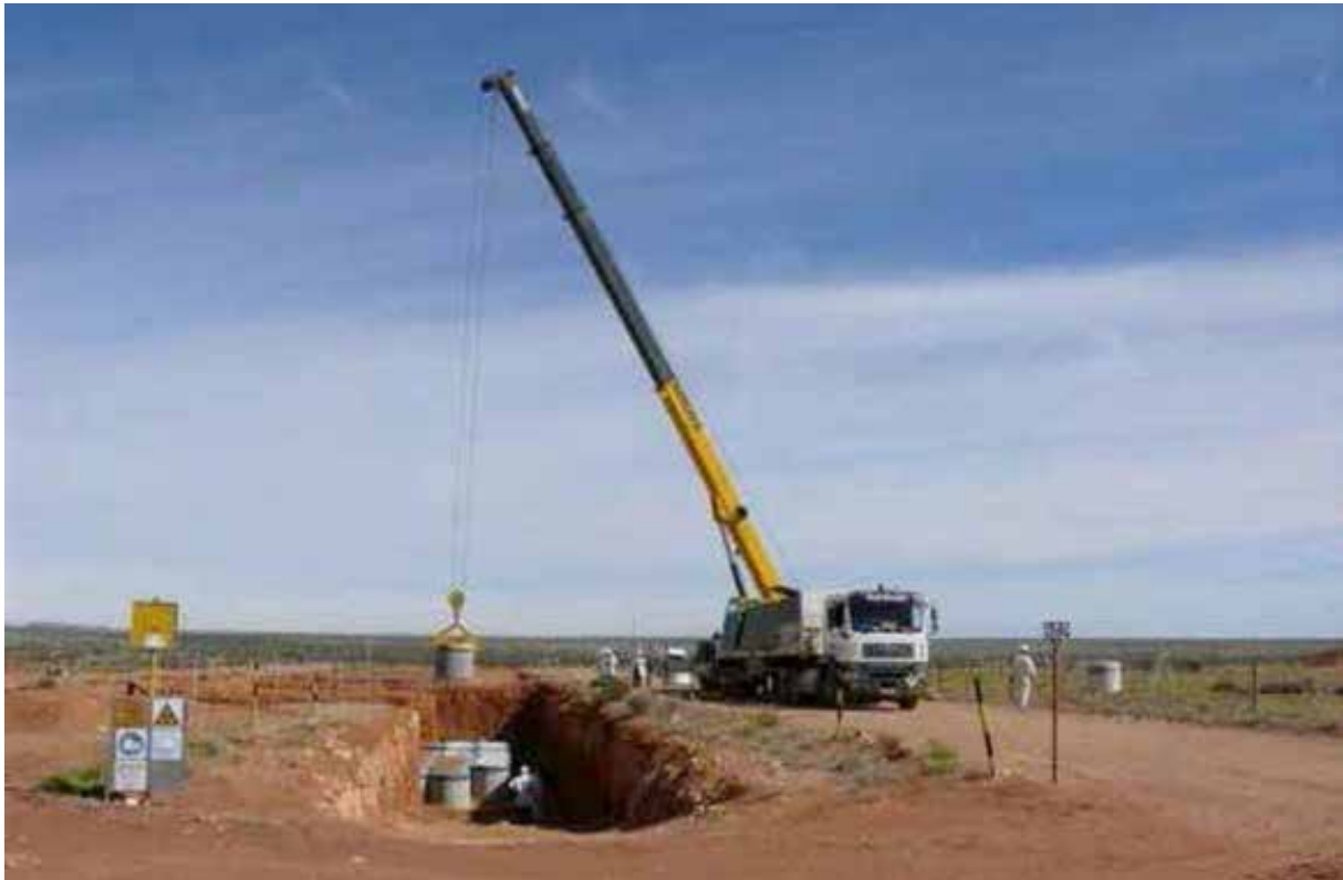
Figure 33: Concrete waste packages being placed into a disposal trench at Vaalputs
