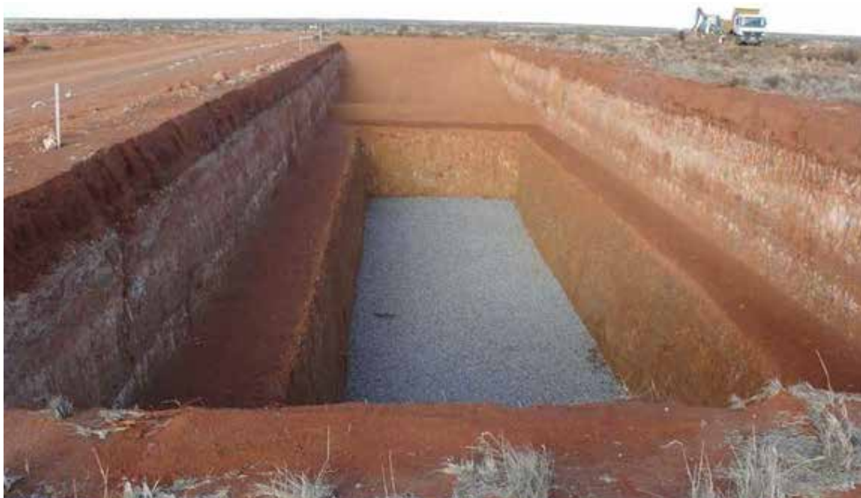
Figure 35: LLW disposal trench at Vaalputs
