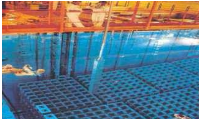
Figure 6: Used fuel pool at Koeberg
