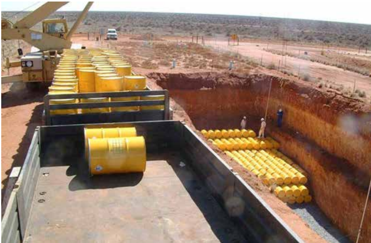
Figure 36: LLW metal containers being emplaced in a disposal trench
