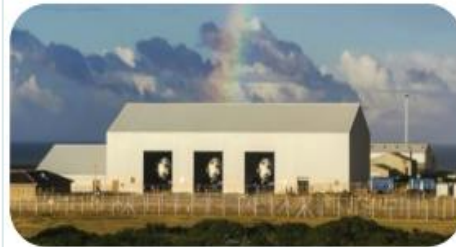
The storage facility housing the replacement steam generators.
