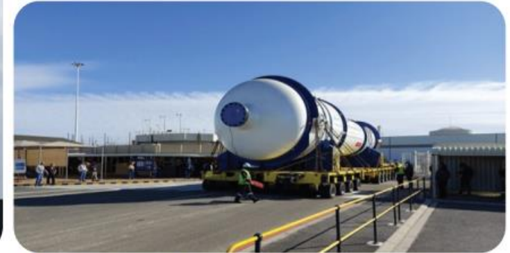
The arrival of one of the six replacement steam generators.
