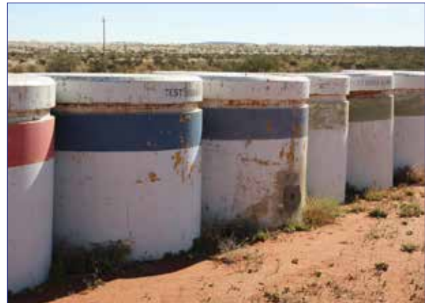
Concrete drums containing radioactive waste
