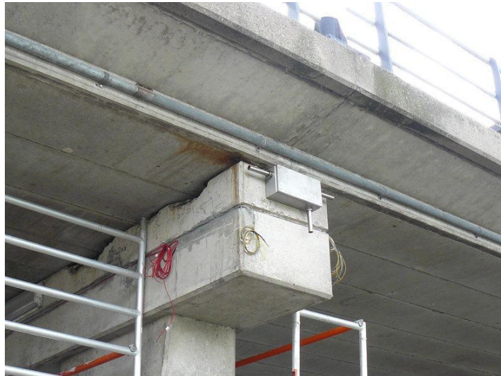
Figure 7: Reinforced cross beam with slots cut
