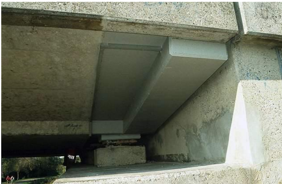
Figure 5: Post-tensioned end beam with conductive coating CP applied
