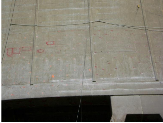
Figure 5-6. Slotted Titanium Ribbon Mesh Anode System and Probe Titanium Anode System
