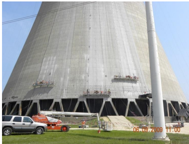
Figure 5-7. Installation of an Impressed Current System on a Hyperbolic Cooling Tower
