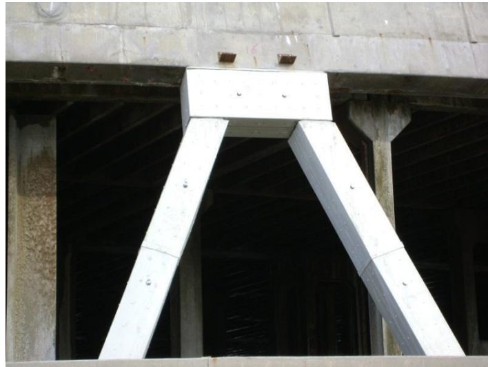
Figure 5-8. Lif jacket System for Lintel Beam and Support Columns
