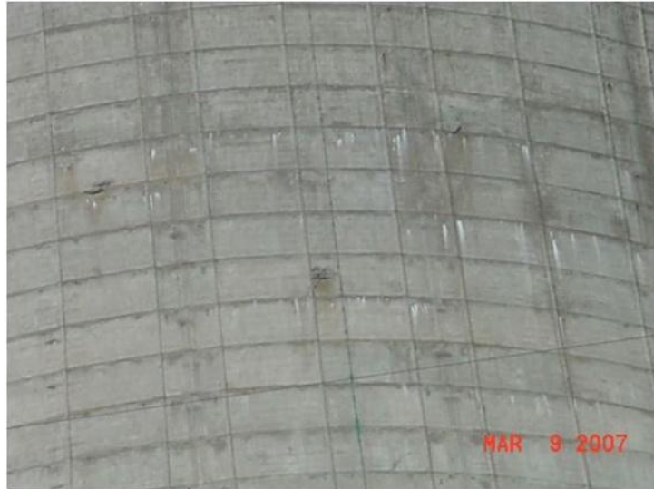
Figure 9: Slotted Titanium Ribbon Mesh Anode System and Probe Titanium Anode System ( [REDACTED] )
