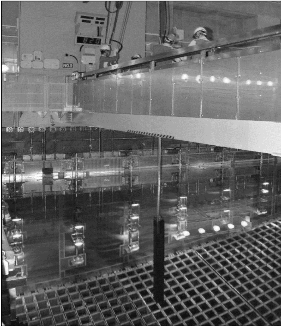
Figure 22: Fuel assembly being moved into storage in a spent fuel pool similar to Koeberg
