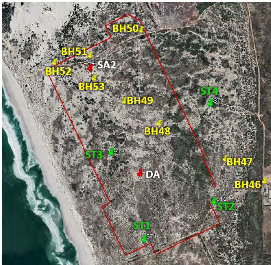
Figure 9-64. Locations of SRK boreholes (BH), MASW/MAM surface arrays (DA, SA2), and CGS boreholes (DA, SA2, ST).
