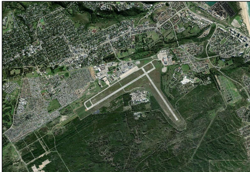
Figure 5.7.2 Aerial Photograph of CDSIA
